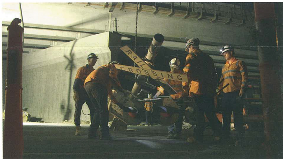
Workers dismantling the Melton Highway boom gates
