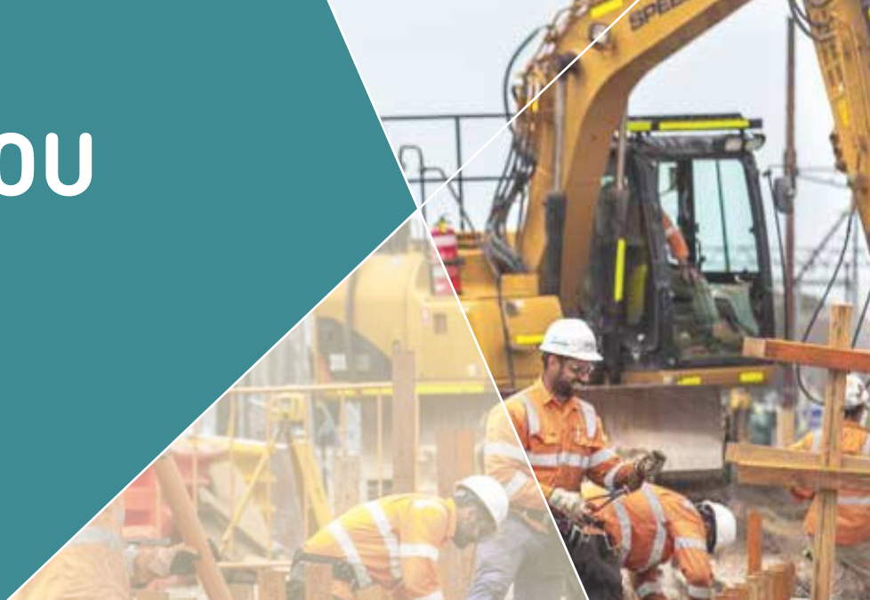
Major works continue in 2020 in Cheltenham and Mentone
