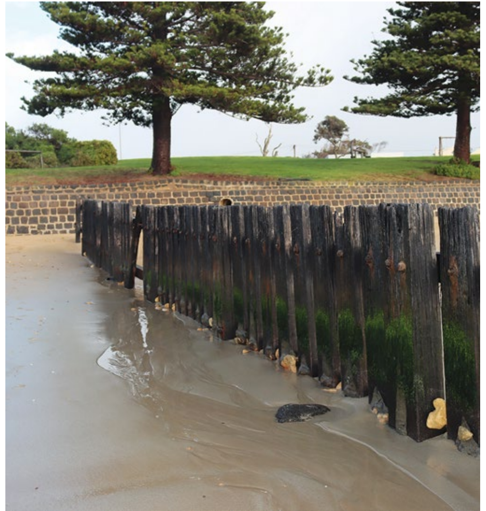
Groynes at Torquay Front Beach.
