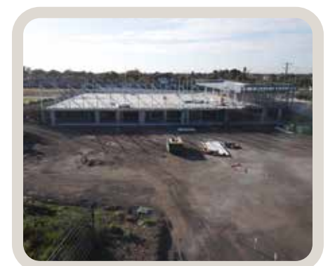
11 May 2020 Constructing level 2
