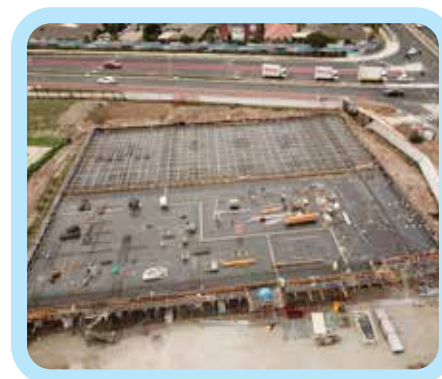
20 March 2020 Constructing level 1
