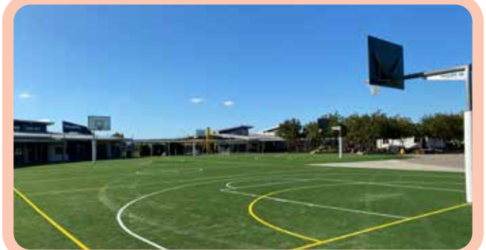
Resurfaced basketball court
