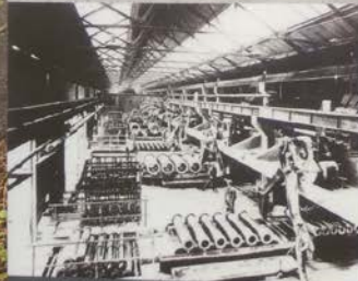
Photo: The Pipe making process, Museum of the Living West
