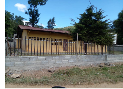
The new fence & gate
