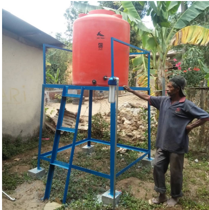
One of 4 new water tanks: primary school, maternity centre, kindergarten, junior high school.
