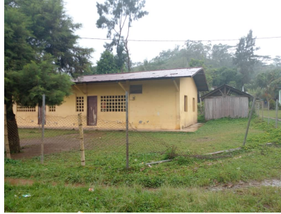
The dangerous wire fence
