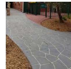
4. STENCILLED CONCRETE PATH
