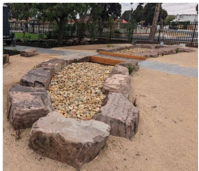
BUILDER TO ENSURE LARGE ROCKS ARE INSTALLED ON THE PERIMETER OF DRY CREEK. ENSURE FLAT SURFACE AS PER PHOTO.
