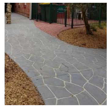
4. STENCILLED CONCRETE PATH
