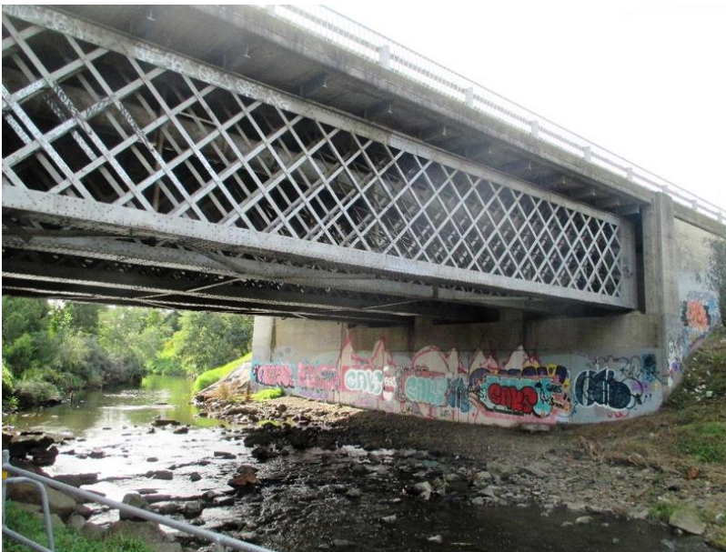
Figure 1.3: Bell Street Bridge Today
