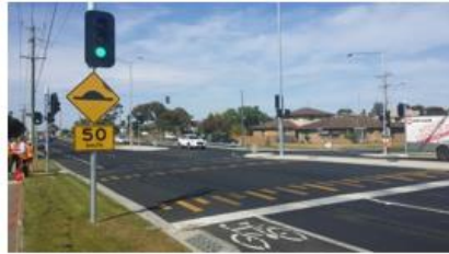
1: Raised Safety Platform
