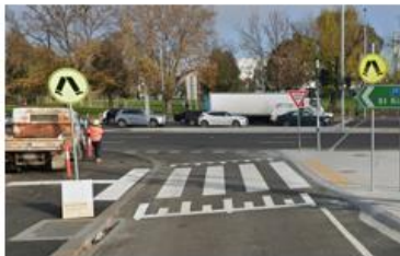
4: Raised Crossing on Slip Lane
