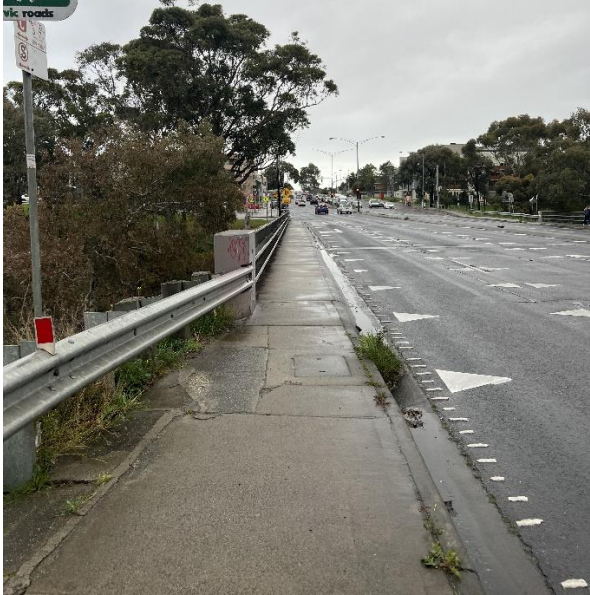
Southern footpath in south-east aspect facing west
