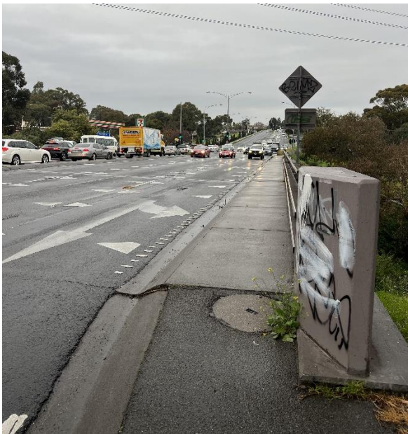
Bell Street southern side facing east
