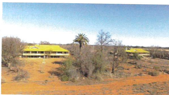
Homestead and manager's residence at Nulla Nulla outstation.
