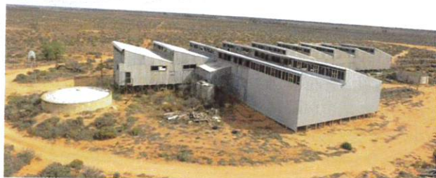
The famous saw-toothed roof on woolshed at Nulla Nulla Built 1920.
